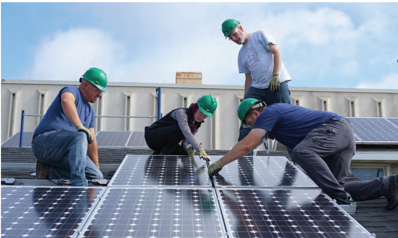
Participants put the finishing touches on a solar energy installation during a Center for Renewable Energy Advanced Technological Education's (CREATE) Faculty Energy Institute. (See page 30)
