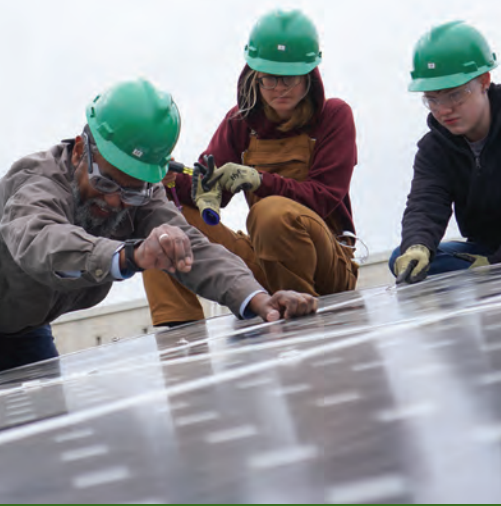
Students install solar panels on the pitched roof that is part of the outdoor lab at Madison Area Technical College.
